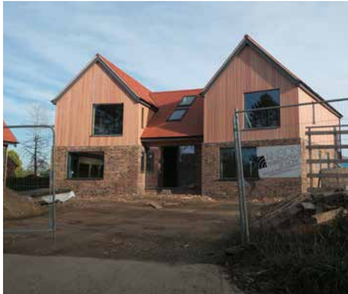
Figure 49: New houses using traditional materials (naturalised wood, red brick, and pantile roofing) in a contemporary style.
