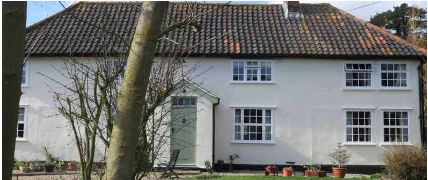
Figure 47: Building displaying a consistent traditional window style and shapes across the main elevation.
