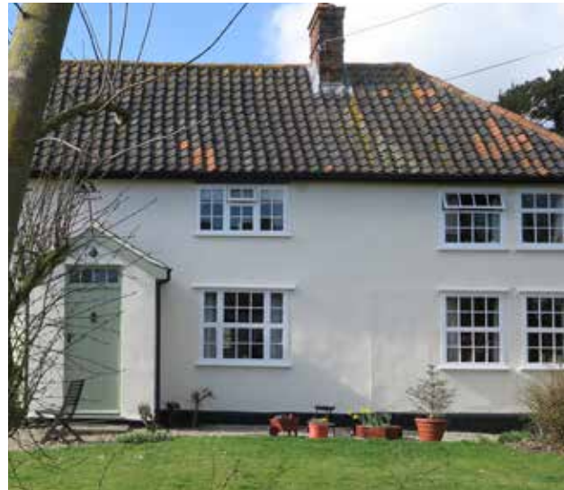
House with off-white rendered walls, pantile roofing, and gabled porch.
