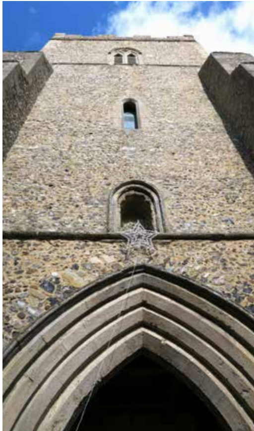
Gothic church tower with flint infill and stone quoins and arches.
