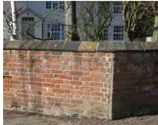
Red brick boundary wall.
