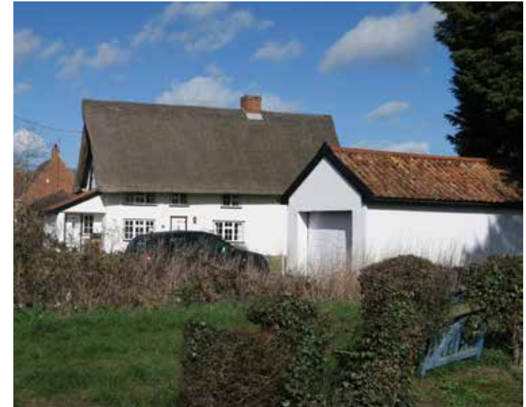
Figure 40: Side garage (right) with local building materials.
