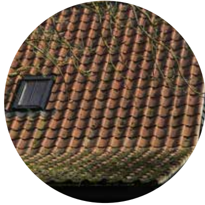
CLAY PANTILE ROOF
