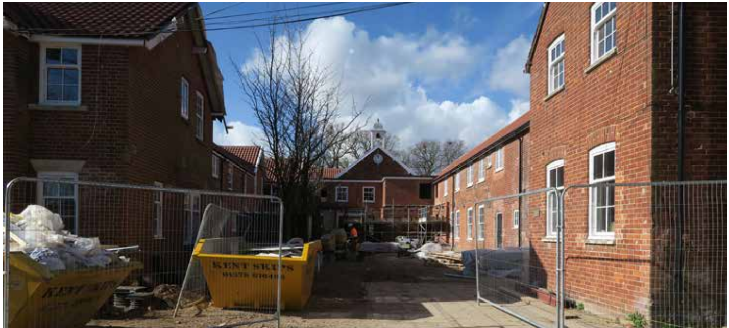
Figure 26: The old reformatory in the Kerrison Conference Centre - the gabled corner pavilions at the end of each wing create a sense of arrival and frame the view towards the central element of the courtyard.
