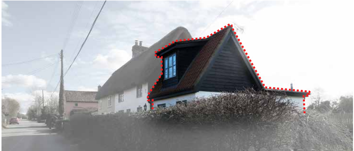
Figure 36: Successful contemporary side extension on The Street.
