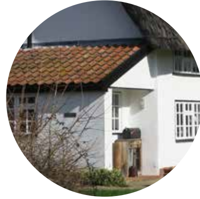
SIDE EXTENSION WITH LEAN-TO ROOF
