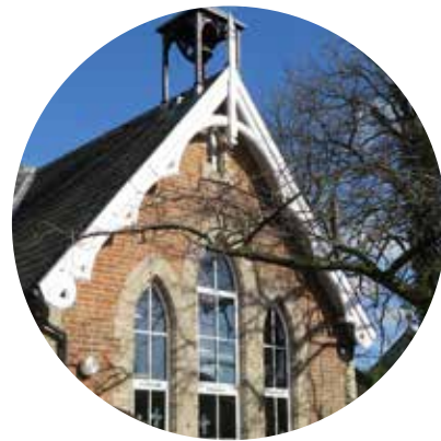
DECORATIVE BARGE BOARD
