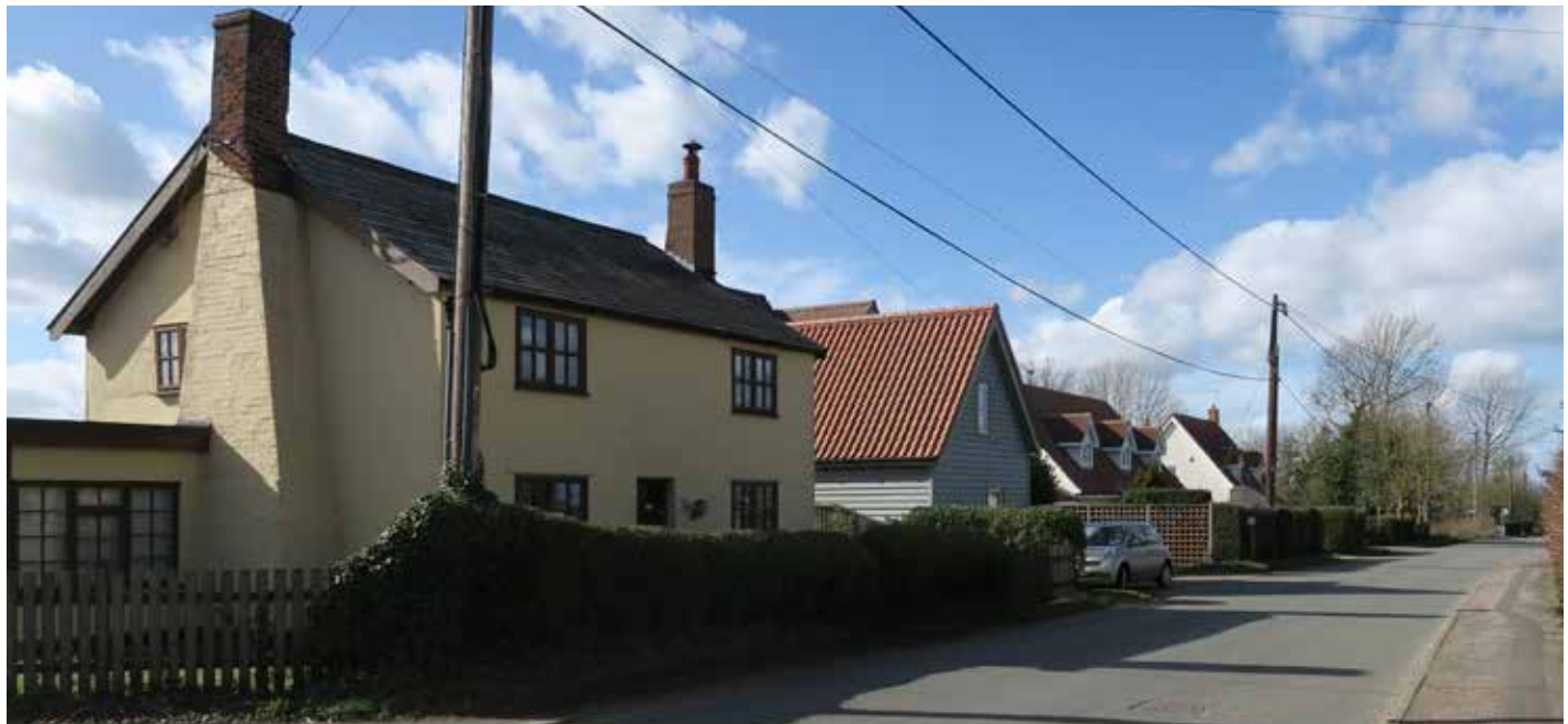
Figure 35: Houses on The Street showing a dynamic roofline with a diversity of roof orientations, pitches, and materials (slate, pantile, and plaintile).
