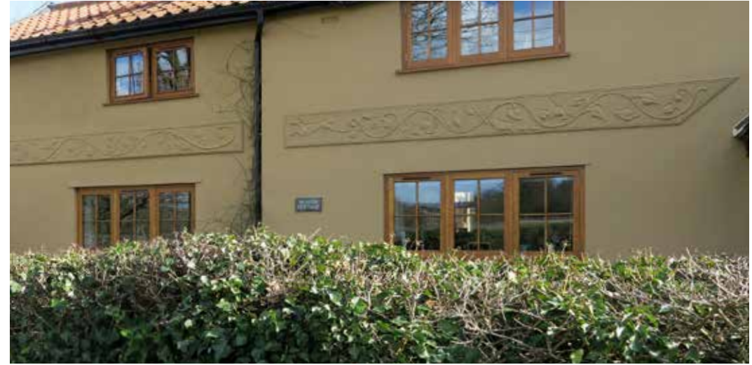
Yellow-rendered façade with pargetting and landscaped boundary treatment.
