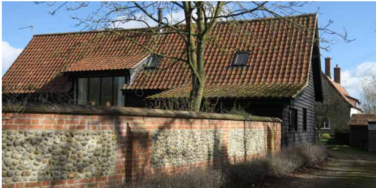
Figure 51: Renovated building and wall using traditional materials such as flint, red brick, black weatherboarding, and pantile roofing.
