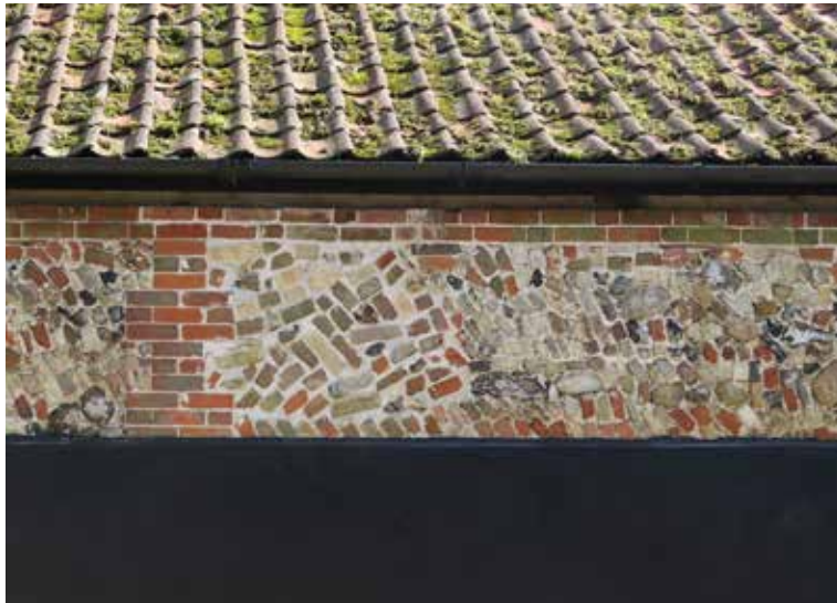
Wall with red brick trim, polychrome brick infill, and pantile roof.
