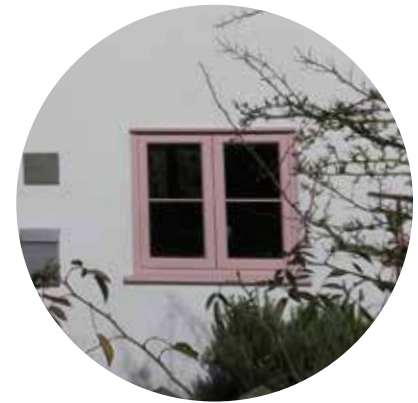
PAINTED WINDOW FRAMES
