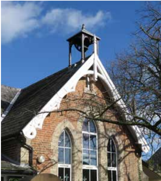
Primary school bicolour brick gable with lancet windows and decorated barge board.
